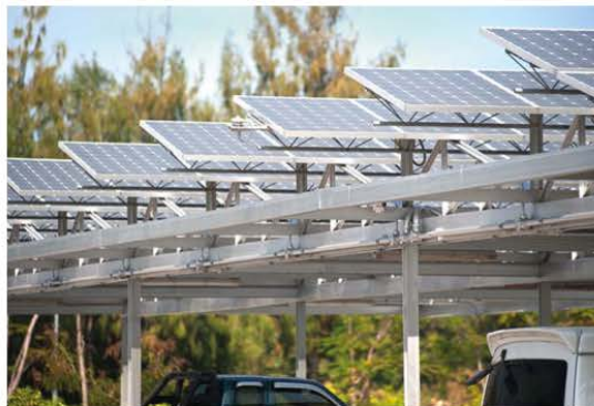
Example of solar carport which will get free energy from the sun, but also incorporate shade protection for the carpark as a bonus
