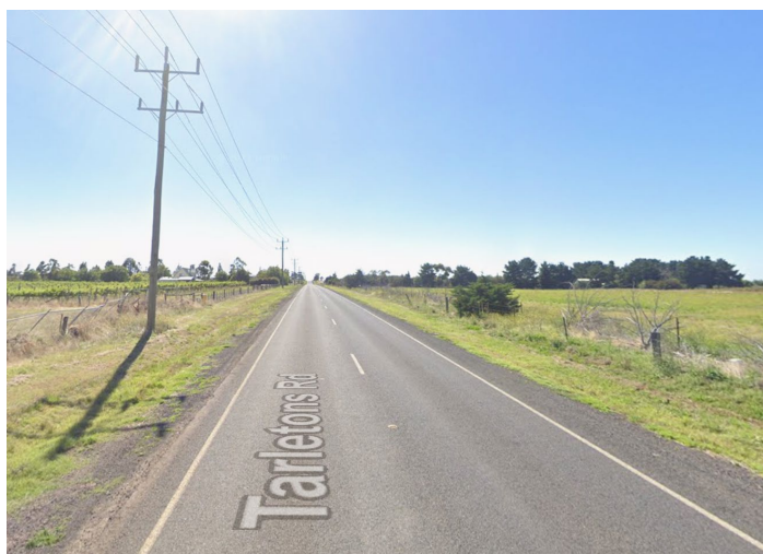
Figure 3 - Tarletons Road Sealed Section
