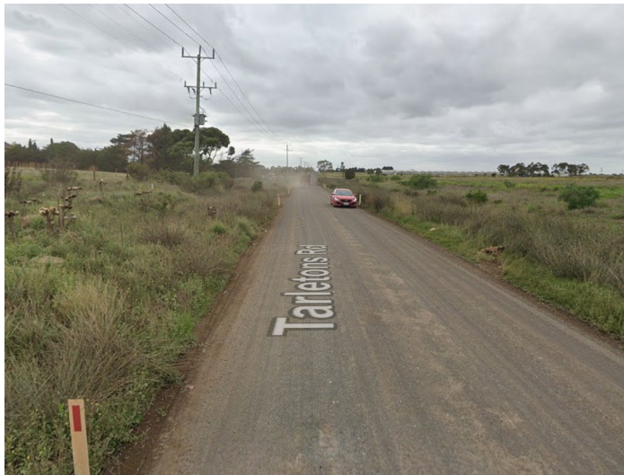
Figure 4 - Tarletons Road - Unsealed Section
