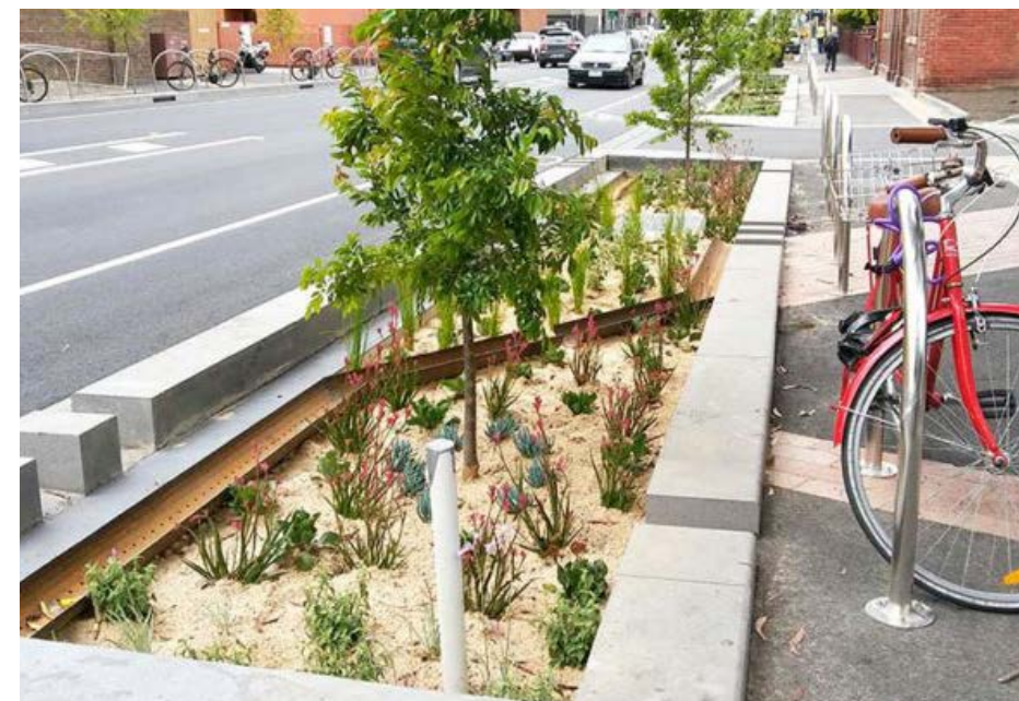
On-street rain garden and stormwater attenuation will help add amenity to the streetscapes
