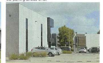
Car parking at side of lot
