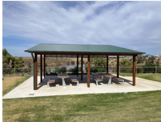
Double skillion roof shelter as installed in Weir Views
