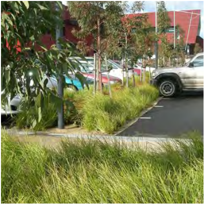
Water Sensitive Urban Design techniques in at-grade car parks, between rows of car parking to treat stormwater before it is discharged from the site and passively irrigate vegetation.
