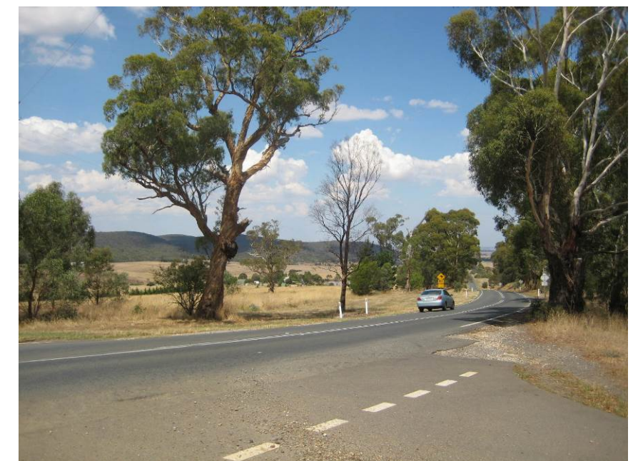
Views along the Diggers Rest-Coimadai Road
