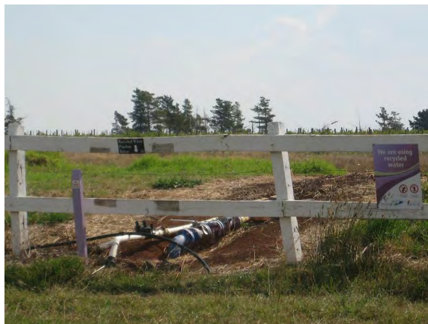
Recycled water pipeline
