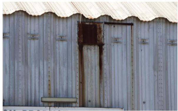
South wall, location of elevator to track
