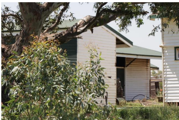
Mid century stable, view from east
