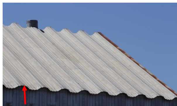
Undulating profile of cladding. Strengthening point with two rows of rivets (indicated).
