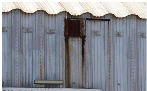
South wall, location of elevator to track
