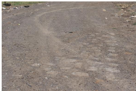
Cobbles to Beattys Road, immediately to the west of Beattys Bridge
