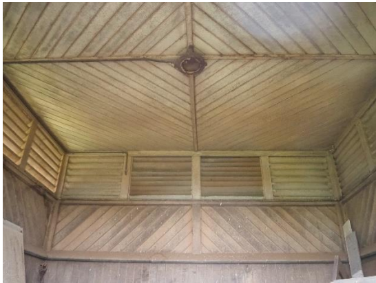
Figure 11 Stallion Box - Interior
