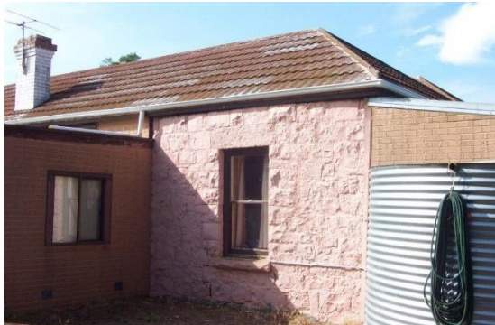
Figure 17 House - North elevation (west end)
