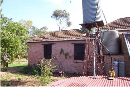
Figure 19 House - West elevation (north end)
