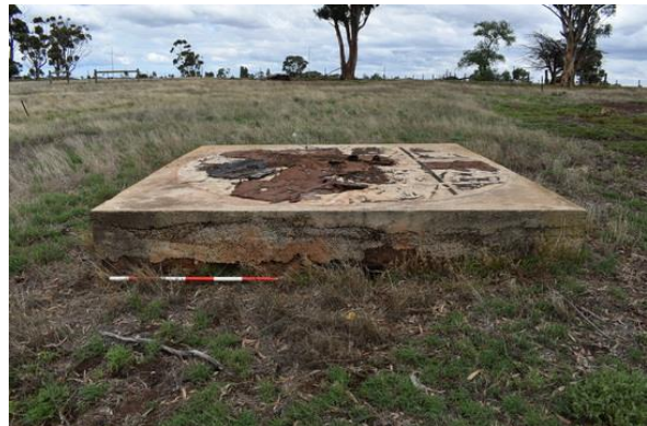
Tank pad constructed of basalt floaters and concrete.
