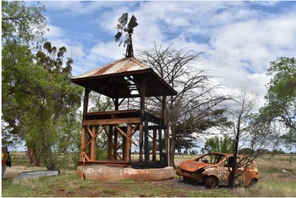
Tank stand, underground brick tank and burnt car.
