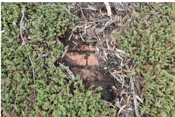
An overgrown portion of brick flooring associated with a former outbuilding.
