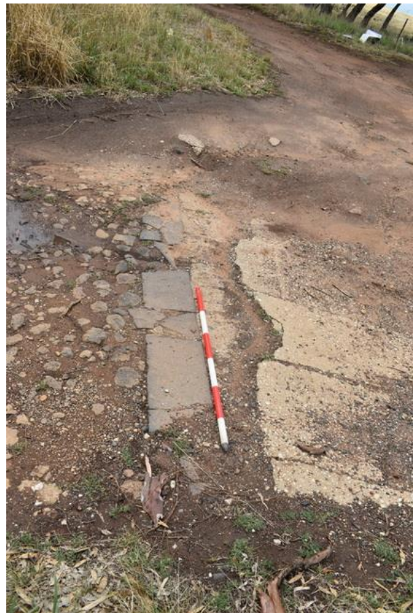
Bluestone blocks and concrete linked to the ford.
