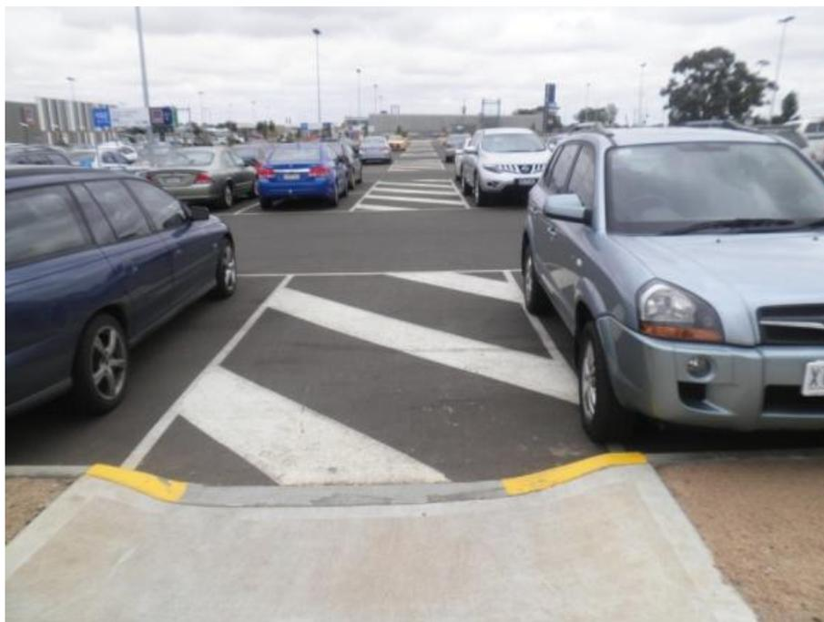
Figure 6 – Pedestrian path not clearly defined and poor sight lines
