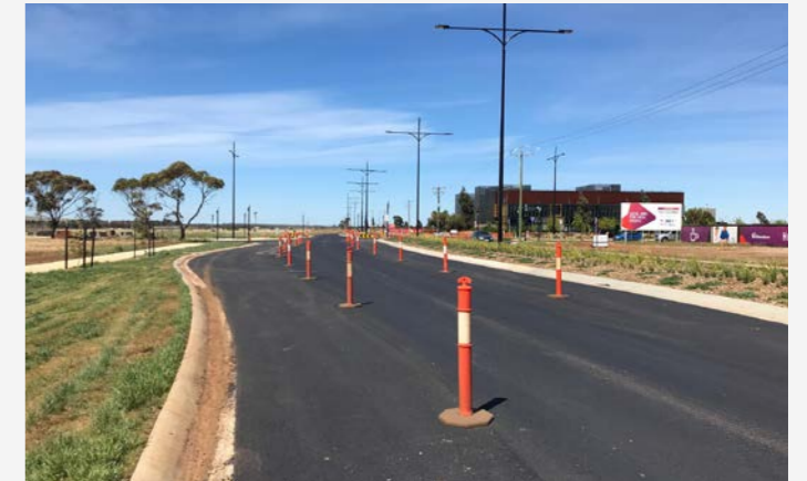
FERRIS & HOLLINGSWORTH DRIVE SIGNALISED INTERSECTION
