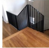
Vertical Metal Balustrade Colour: Woodland Grey Post: 50x50mm SHS Bar: 50x5mm Rail: 20x20mm SHS
