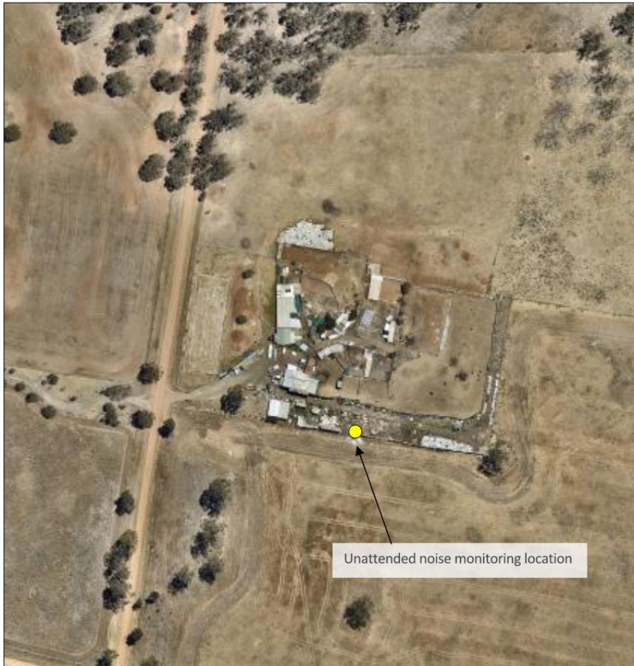
Figure 7: Unattended noise monitoring location
