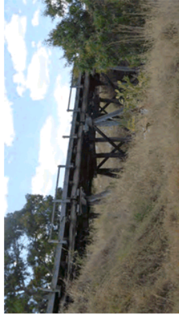
Disused wooden bridge across Toolern Creek
