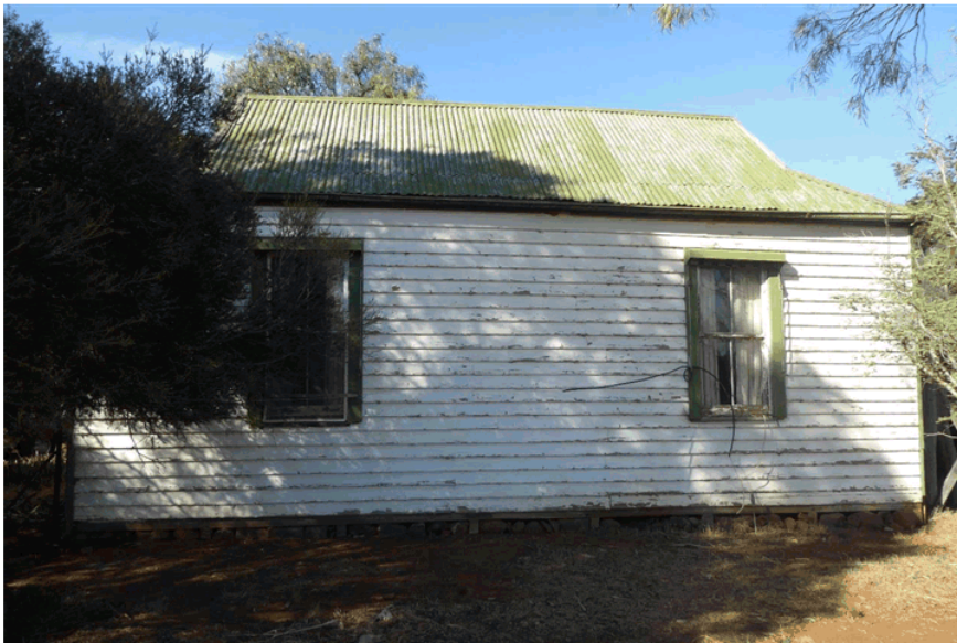
Main gambrel roof section
