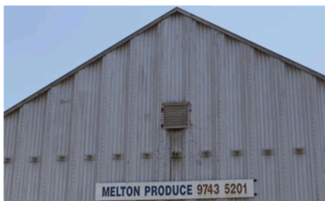
Gable end with vent and band of tie plates below
