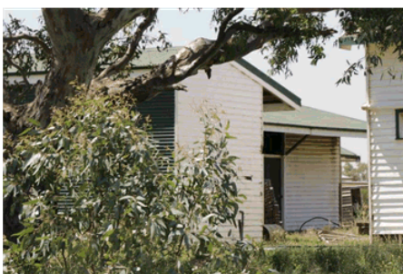
Mid century stable, view from east
