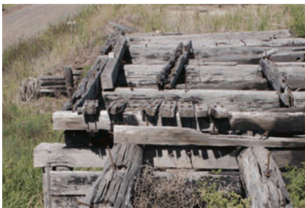
View of bridge from bank with remnant sections of longitudinal deck evident
