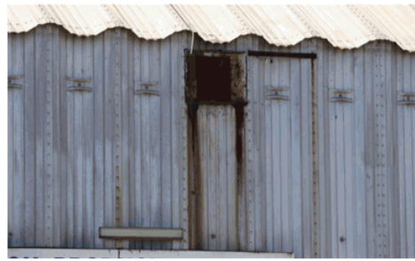
South wall, location of elevator to track
