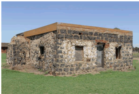
North-east corner of cottage
