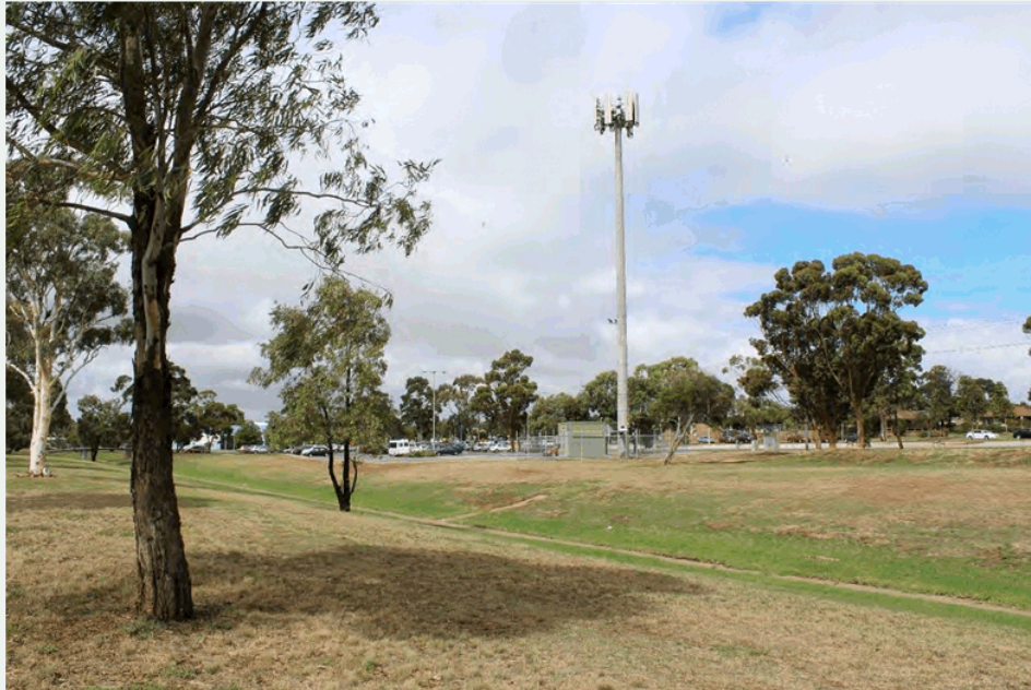
PA2012/3471-2 - Melton Waves Carpark, 206 Coburns Road, Melton West, Vic 3023 – RFNSA No: 3337019
