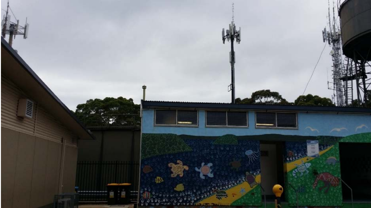
Figure 1 - Two monopoles and a lattice tower.
