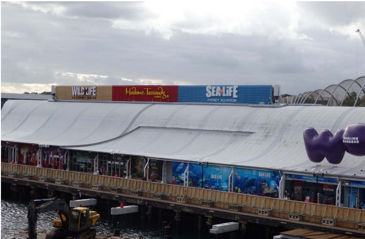
Figure 5 - A rooftop installation that does not break the ridge or overall height of the building.
