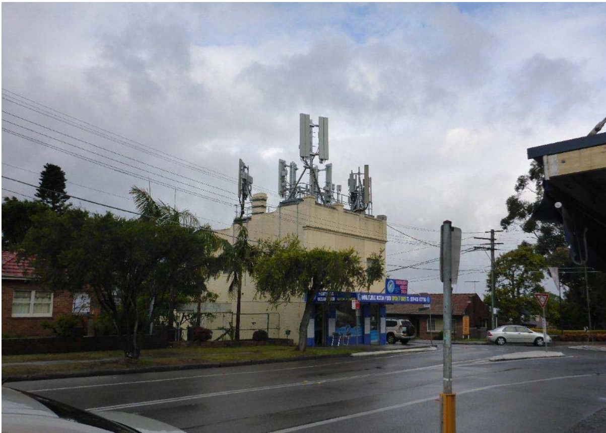
Figure 2 - A rooftop facility overcrowded by facilities.
