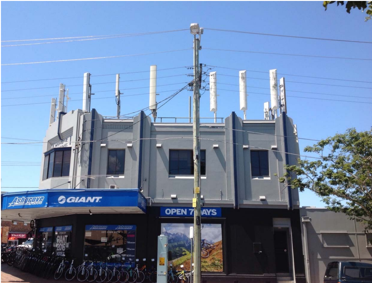
Figure 4 - An obtrusive and overcrowded rooftop.
