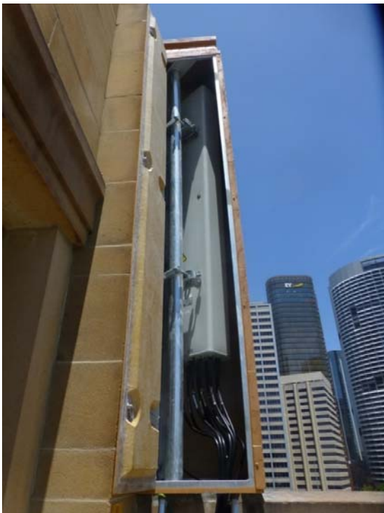
Figure 6 - An example of shrouding/screening on a prominent heritage building.
