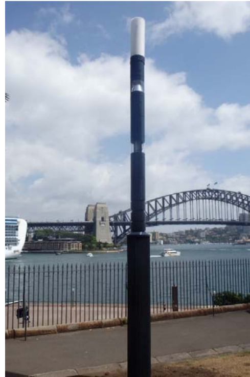
Figure 4 - A small-cell smart pole installation in the Royal Botanic Gardens, Sydney.
