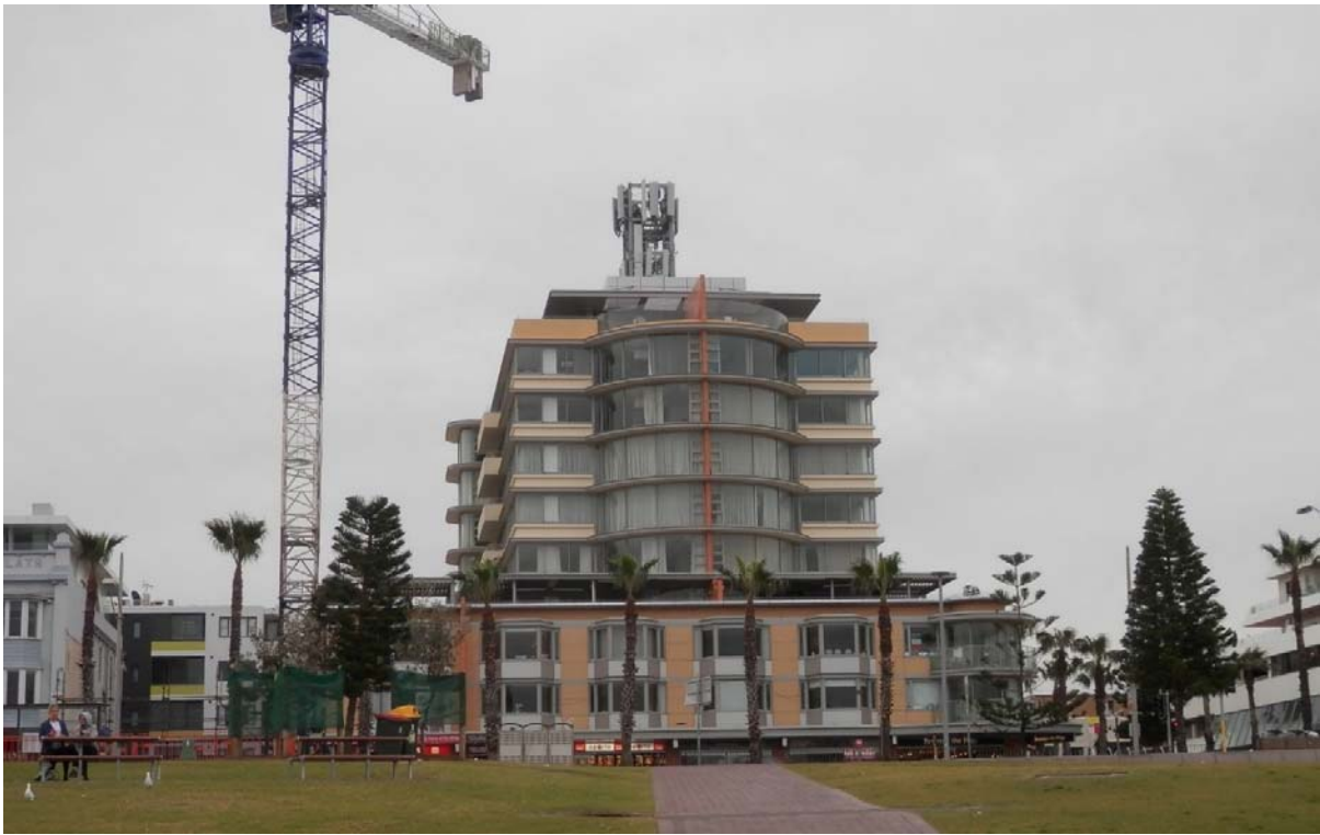
Figure 3 - An obtrusive rooftop facility.
