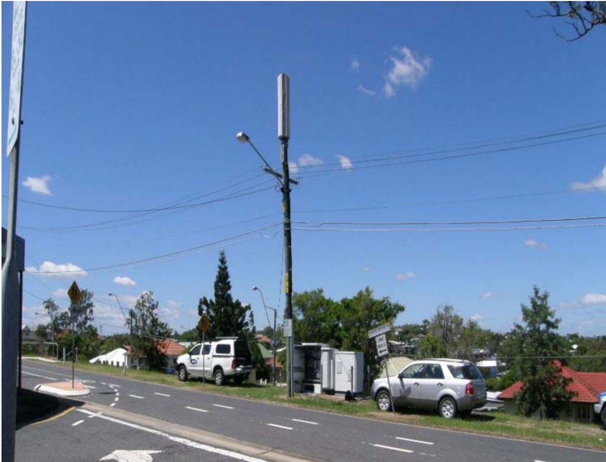
Figure 2 - A co-location facility atop an electricity pole.
