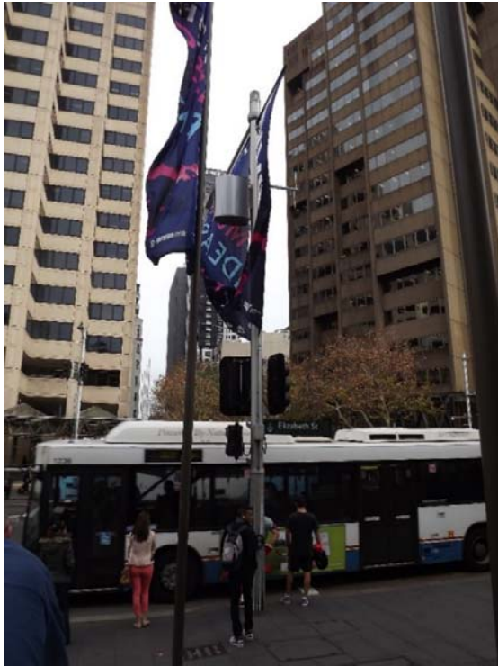
Figure 3 - Small-cell on a smart-pole
