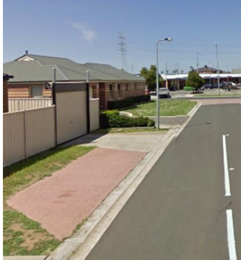
Figure 20 – Light Pole Installed Clear of Parking Bay
