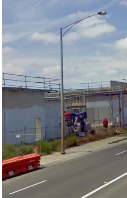
Figure 22 – Light Pole Installed Within Footpath
