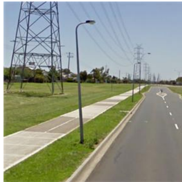
Figure 23 – Light Pole Installed Clear of Shared Path
