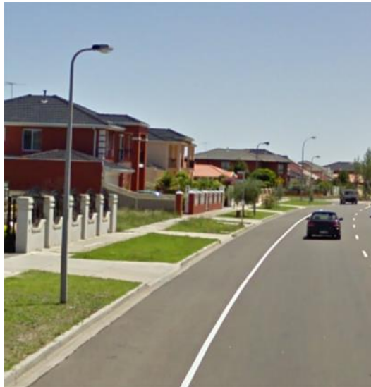
Figure 21 – Light Pole Installed Clear of Parking Lane
