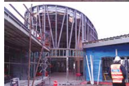
The steel frame is up as Burnside Children's and Community Centre starts to take shape.
