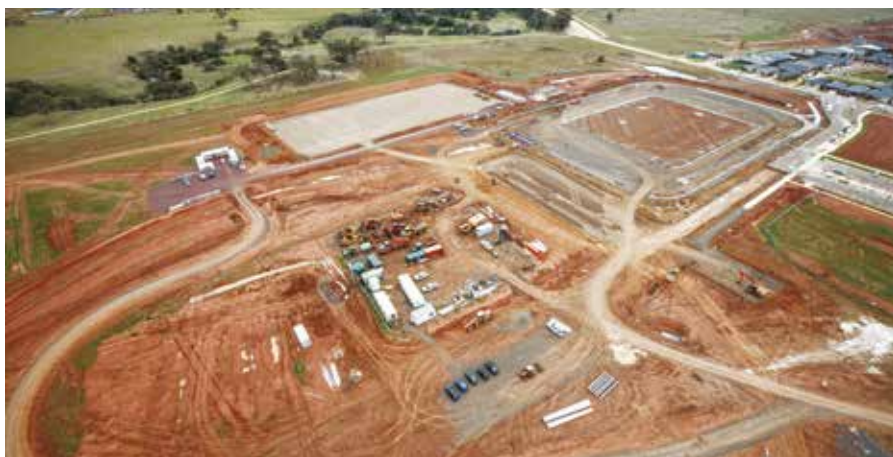
An aerial view showing progress of the Bridge Road Sports Precinct.
