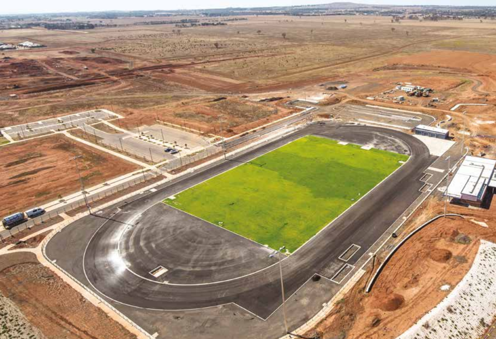
Aerial view of the Bridge Road Recreation Reserve currently under development.
