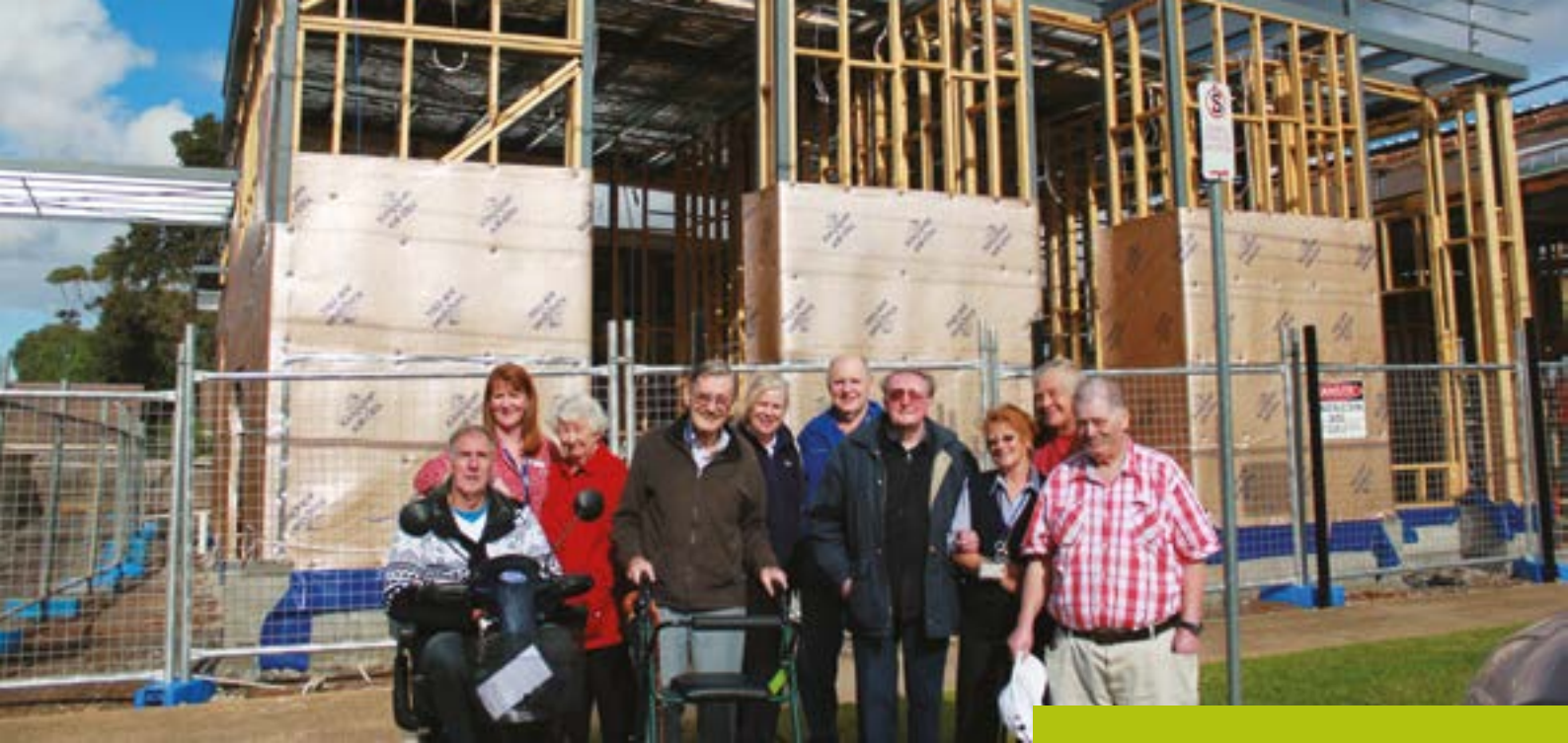
Resident participants and staff at McKenzie Street Aged Services stand proud in front of the facility's extension which is currently under construction.
