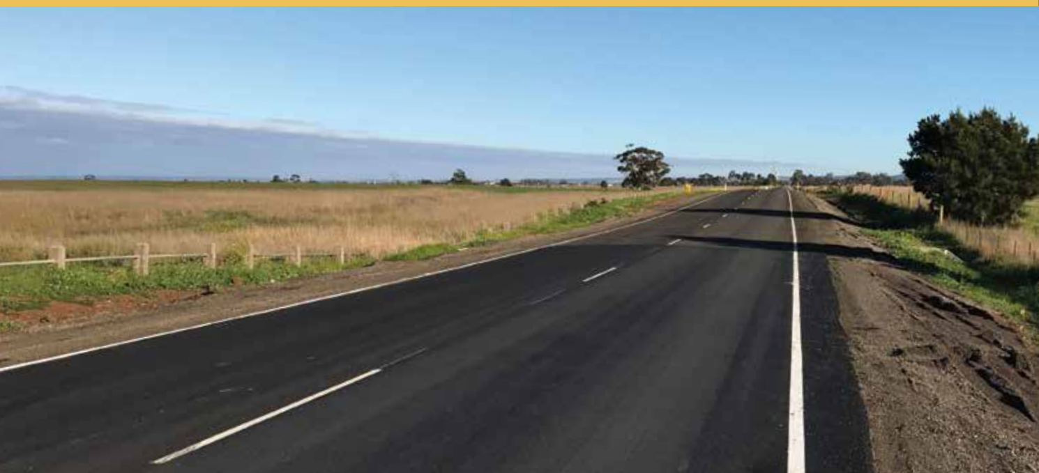
Minns Road construction
