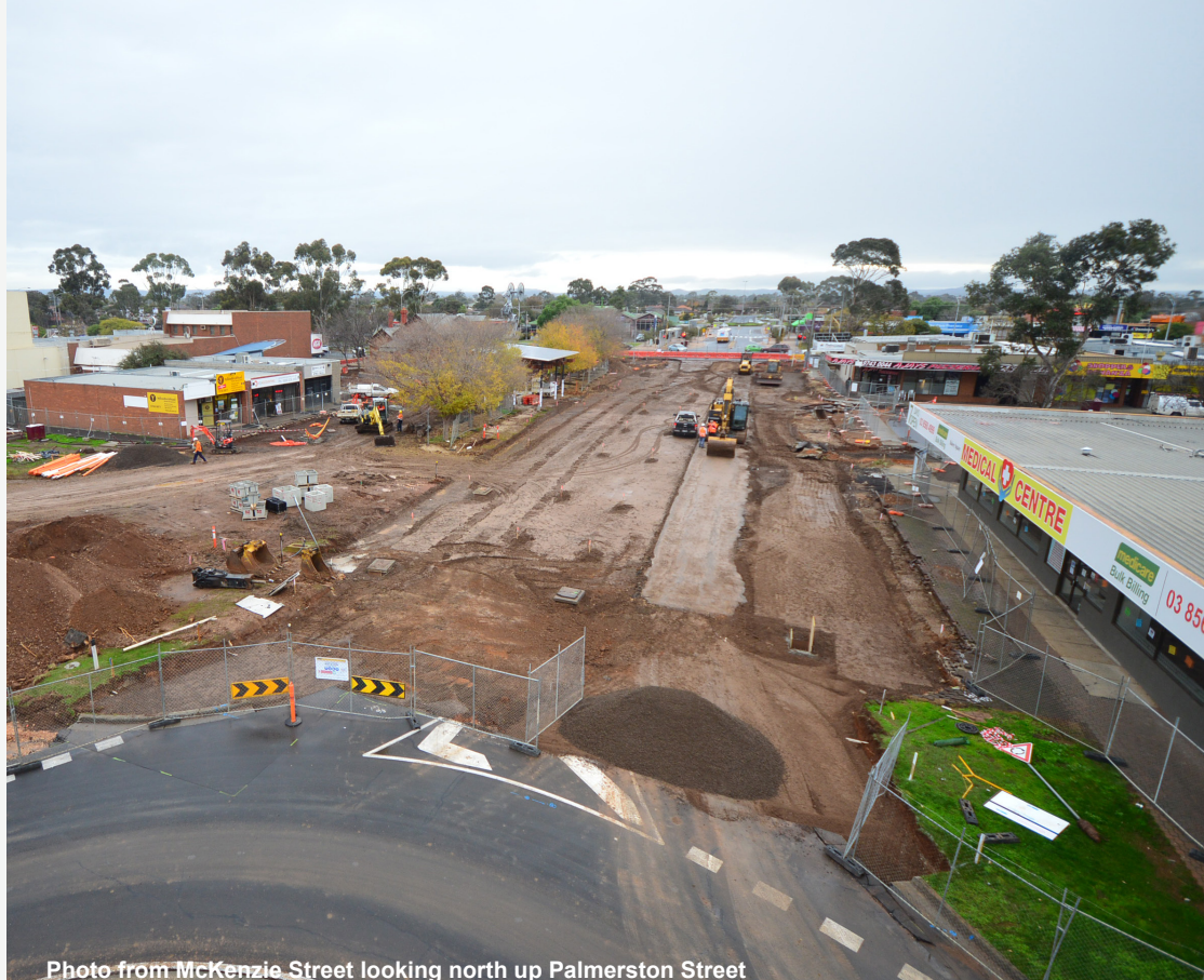
Photo from McKenzie Street looking north up Palmerston Street
