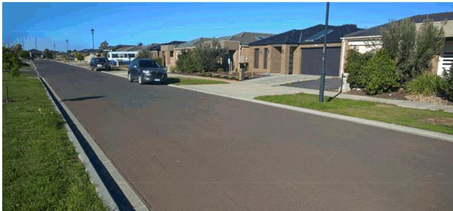
Fieldstone Way, Brookfield – Likely location of raised pedestrian crossing
