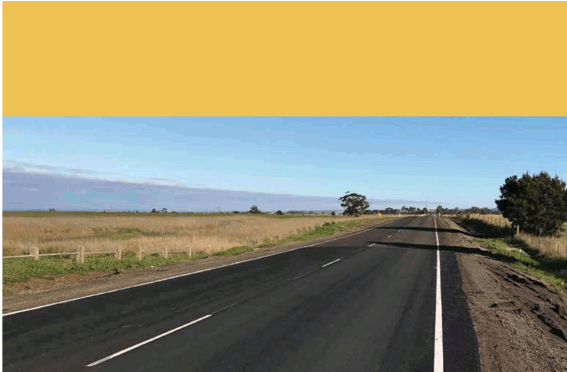
Minns Road construction
