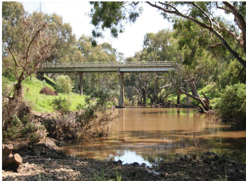
photo 32: greig’s road bridge over the werribee river downstream from melton reservoir
