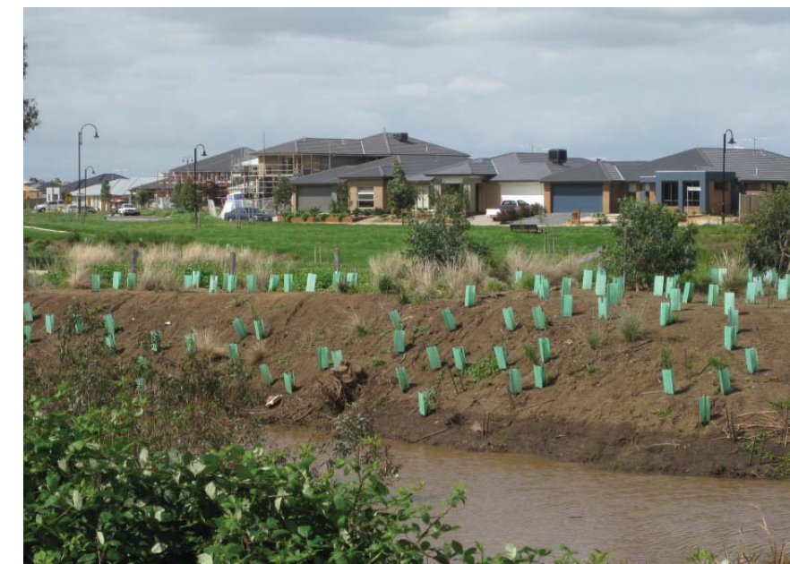
photo 36: rehabilitation works along davis creek, with recent urban development beyond
