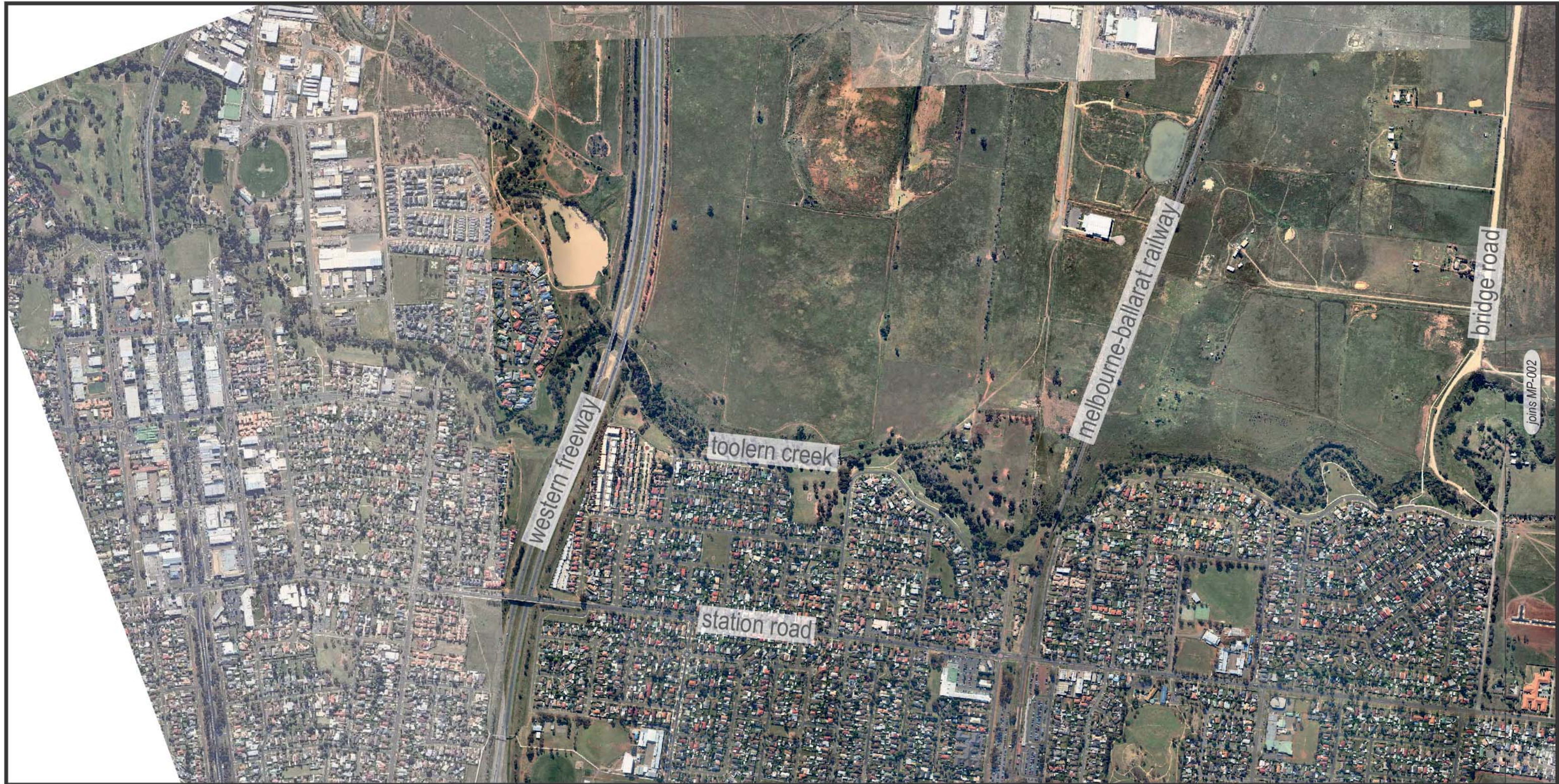
figure 5: existing conditions reach 1
