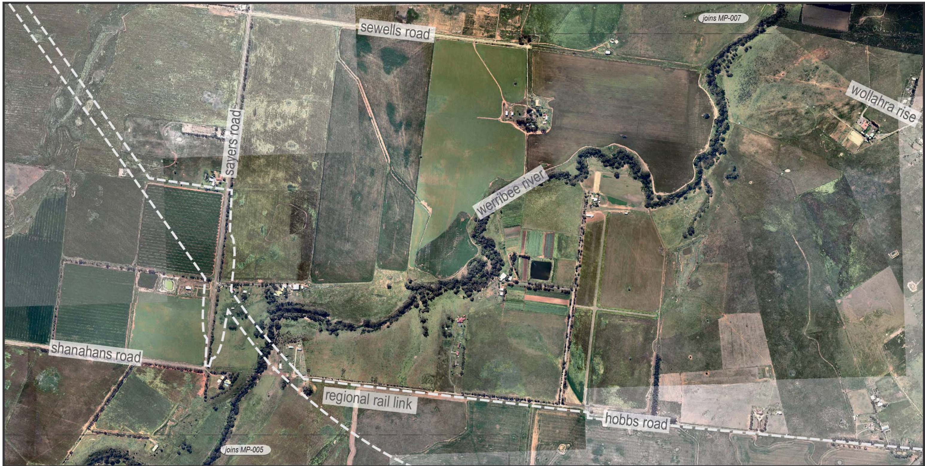
figure 10: existing conditions reach 6
